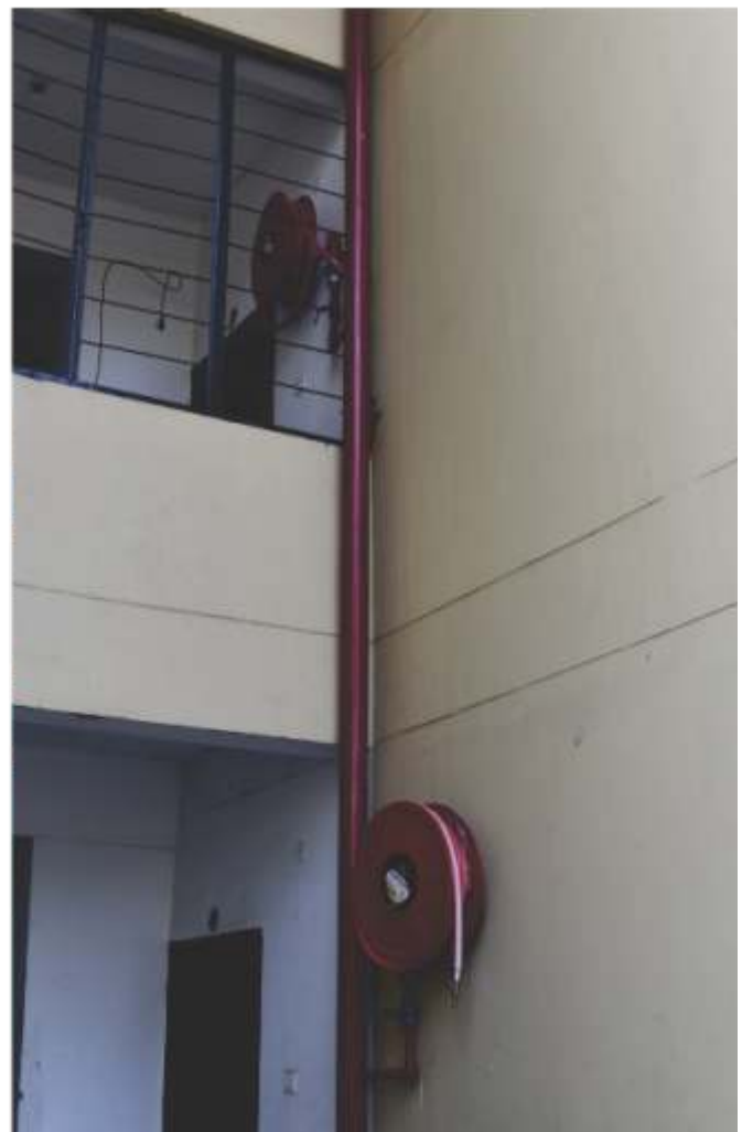
Installation of Fire Hose Reels at Support Staff Colony
